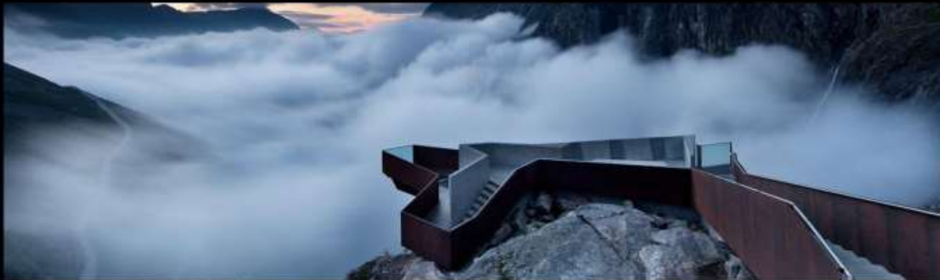
Trollstigen Mountain Lodge, Reiulf Ramstad Architects
